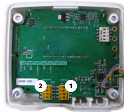
Inside the front housing
